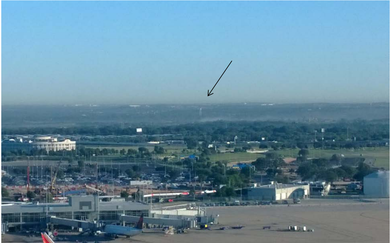
#11 5 N – Travis Co. Corrections (many-legged) Water Tower (Day/Night)
