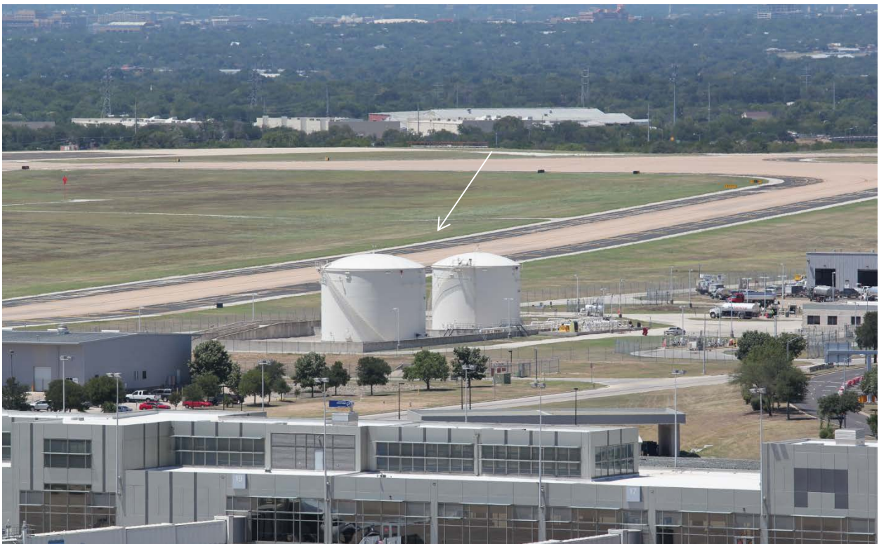
#8 3/4 NW – Fuel Farm Tanks (Day/Night)
