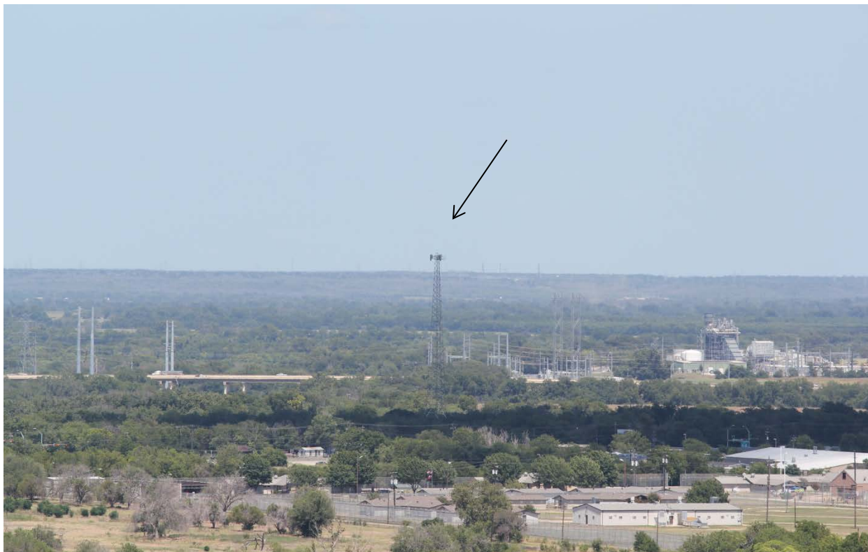
#21 1½ NE – Cell Tower (Day/Night)
