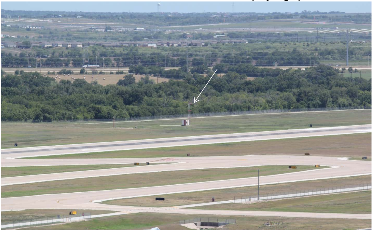
#12 1 SE – RWY 35R Glideslope Building (Day/Night)
