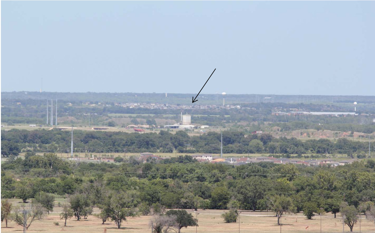
#9 4 NE – Block Building of Texas Industries (Day/Night)
