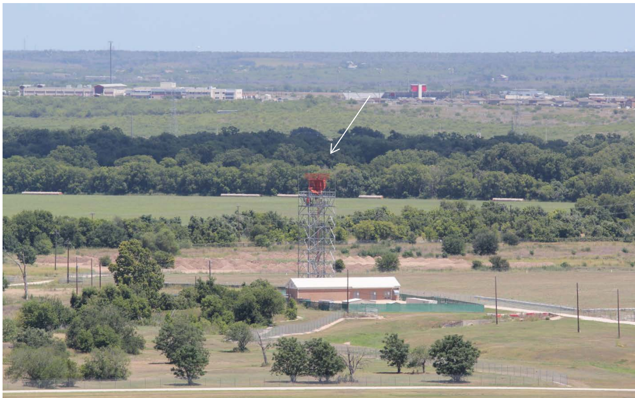
#13 1 E – ASR-9 Radar Antenna (Day/Night)
