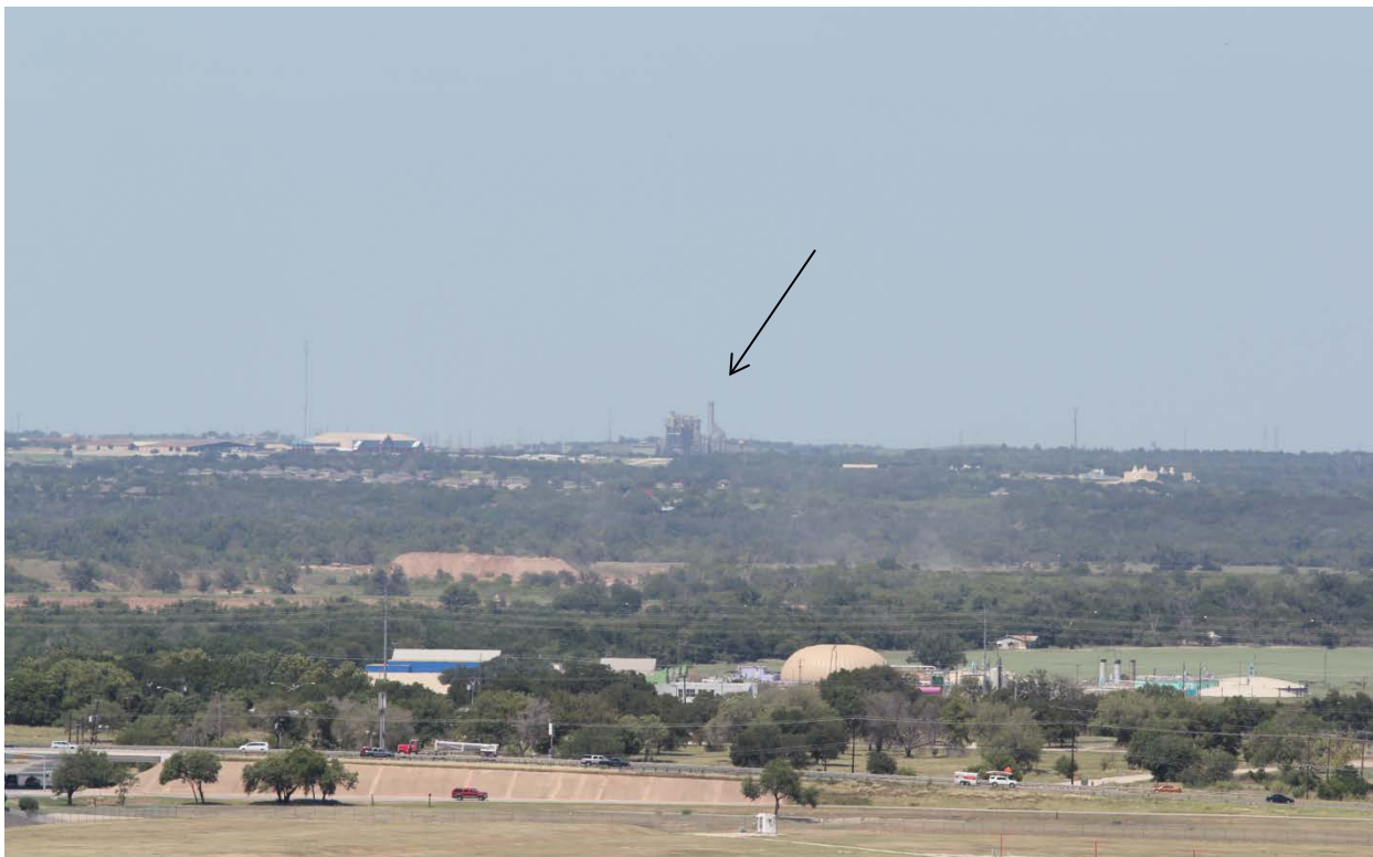
#17 8 N – Decker Creek Power Plant (Day/Night)
