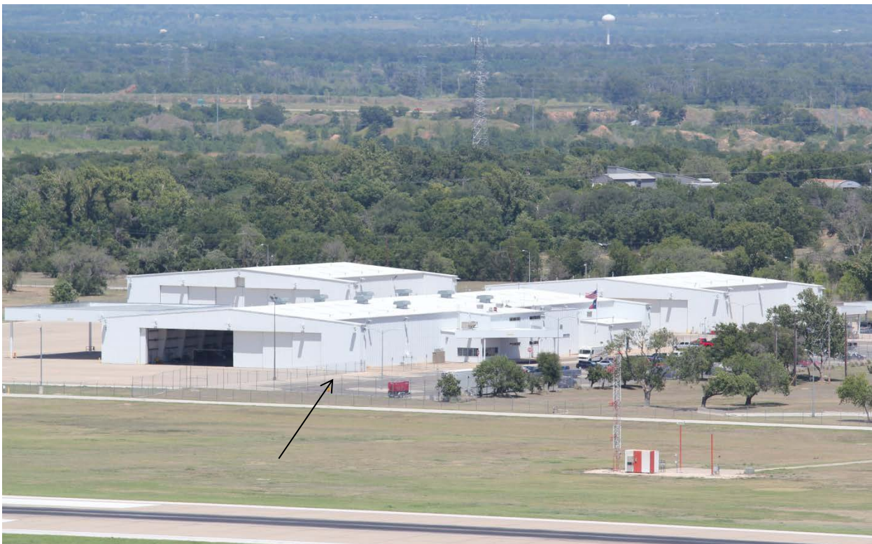
#9 3/4 NE – Nearest Corner of State Ramp Hanger (Day/Night)
