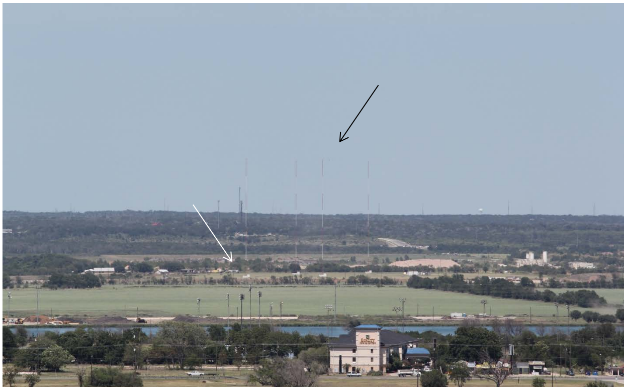
#5 3 NE – KLBJ Antenna Buildings (Day) / Lights (Night)
